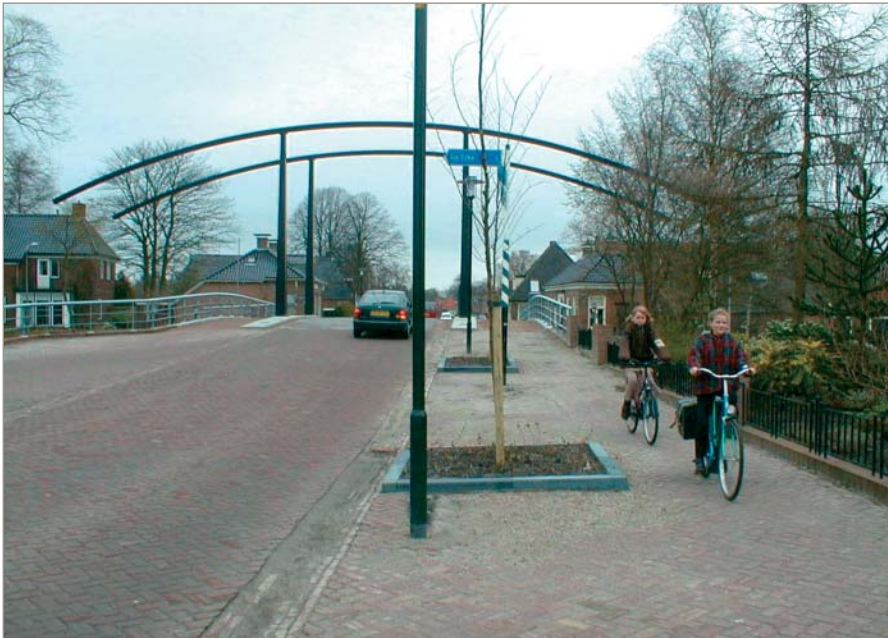
Fig. 9. New urban gateway at Opeinde, Netherlands—once inside the arch, the road surface changes and road markings and kerbs disappear
